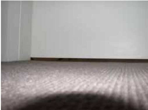
Photo No 19 (fire door base gap >10mm)
