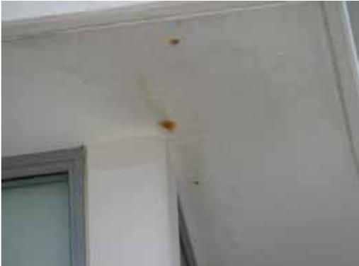
Photo No 63 (Southern corner spalling)
