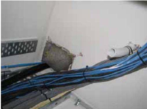
Photo No 16 (carpet underlay filled penetrations)
